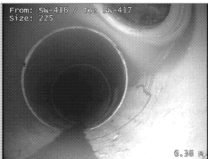
Junction at 1 o'clock, diameter 150mm - Remark: UNKNOWN
