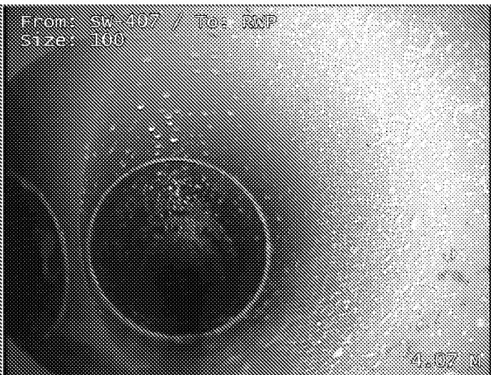
Junction at 11 o'clock, diameter 100mm
