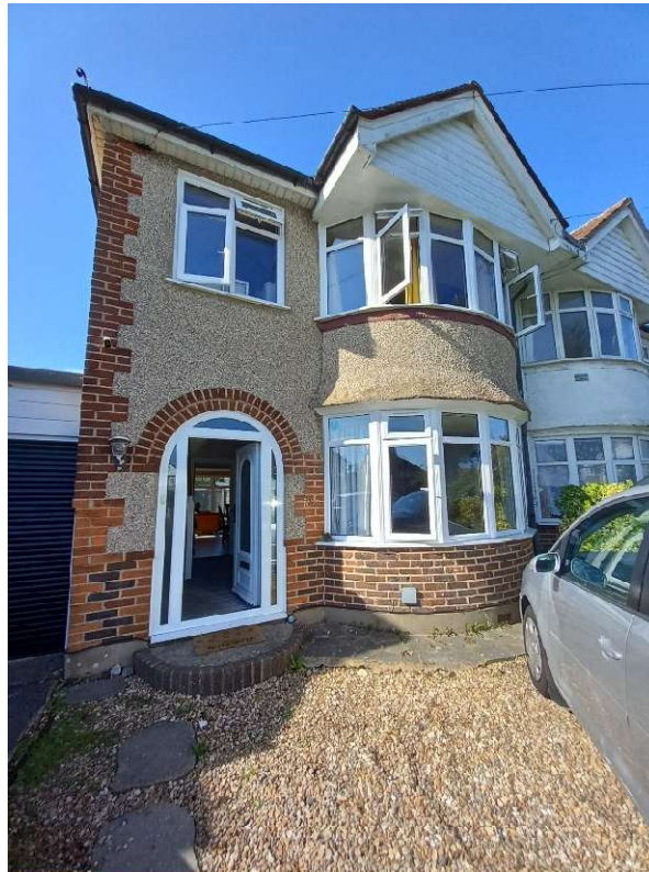
Front elevation of 70 Central Avenue.
