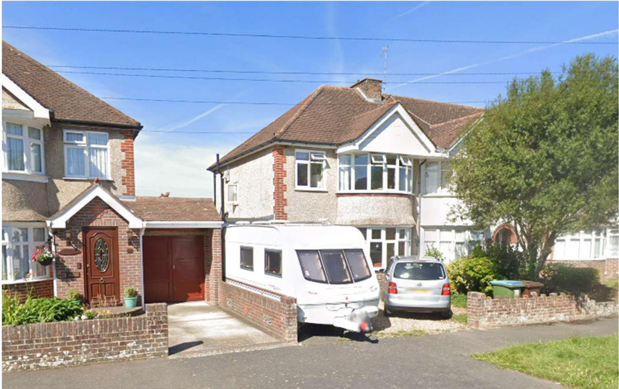
Street view showing 70 Central Avenue in context.
