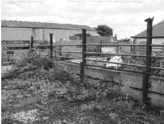
Photo 4. View of the steel tube fencing forming part of one of the old cattle pens within the site.
