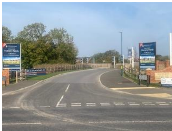
Junction from Chalcraft Lane to Daffodil Avenue with site access in view
