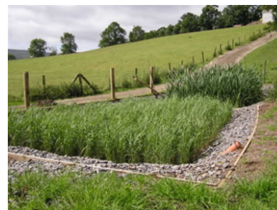
Example of a reed bed system
