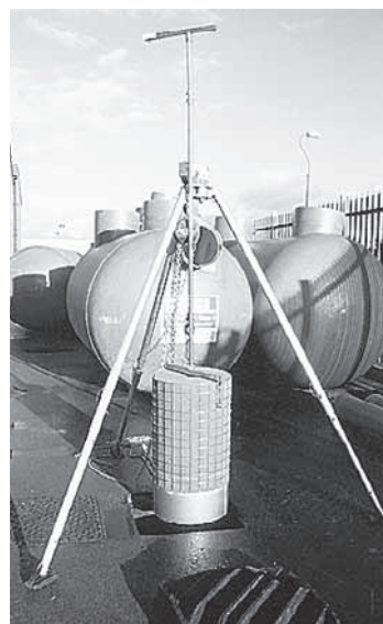
Step 9 – Once the coalescer unit is above ground level, swing it to one side of the manhole for maintenance.
