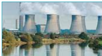
Power stations and electricity sub-stations
