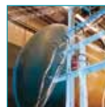
Left: Bristol International Airport SPEL Puraceptor Class 1 full retention separator NS 942 and 'automatic' Econoskim system.
