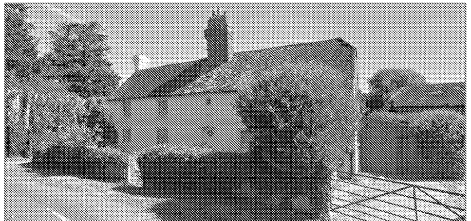
Plate 7 – Looking northeast towards Morells Farmhouse from Lower Bognor Road (image © Google 2020; image date July 2019)
