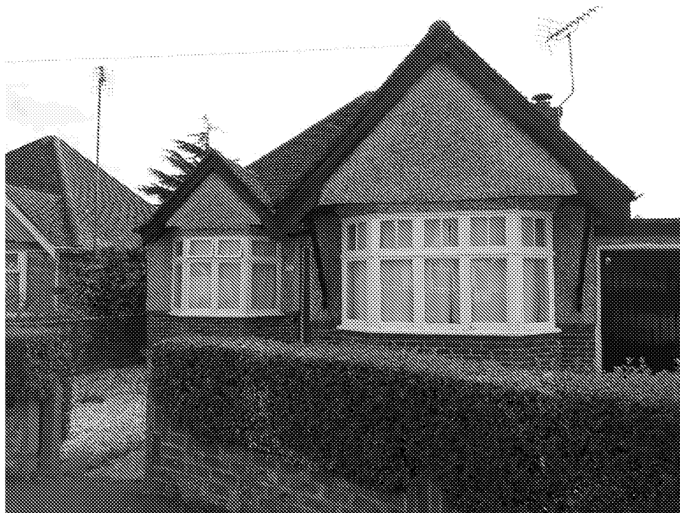
Front of the bungalow (facing east)
