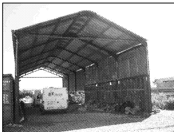
Photograph 12: Open metal barn, south-western elevation
