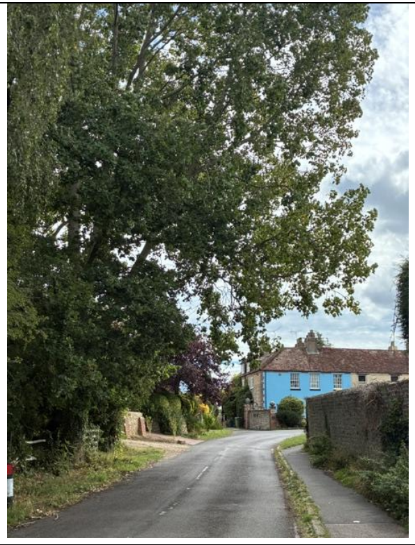
T3 facing south
