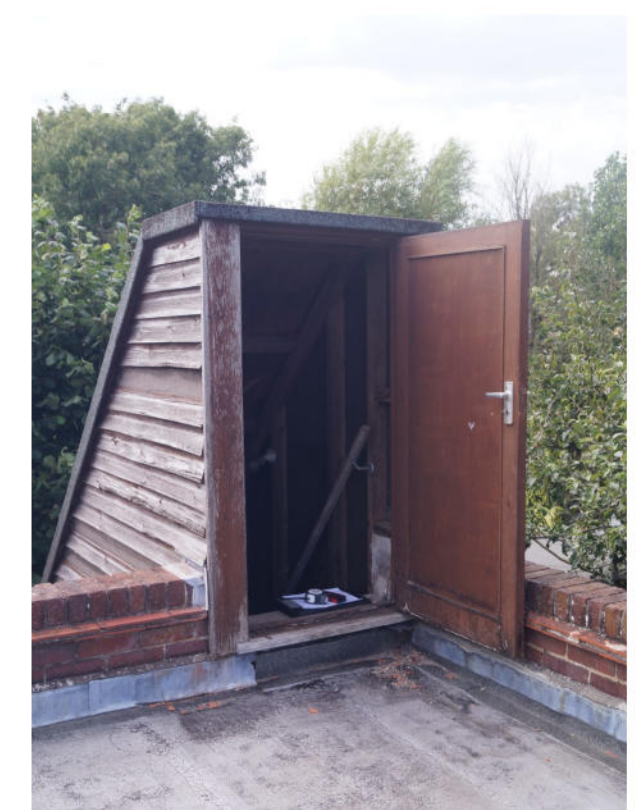
Fig. 5 Barn End - Flat Roof Access
