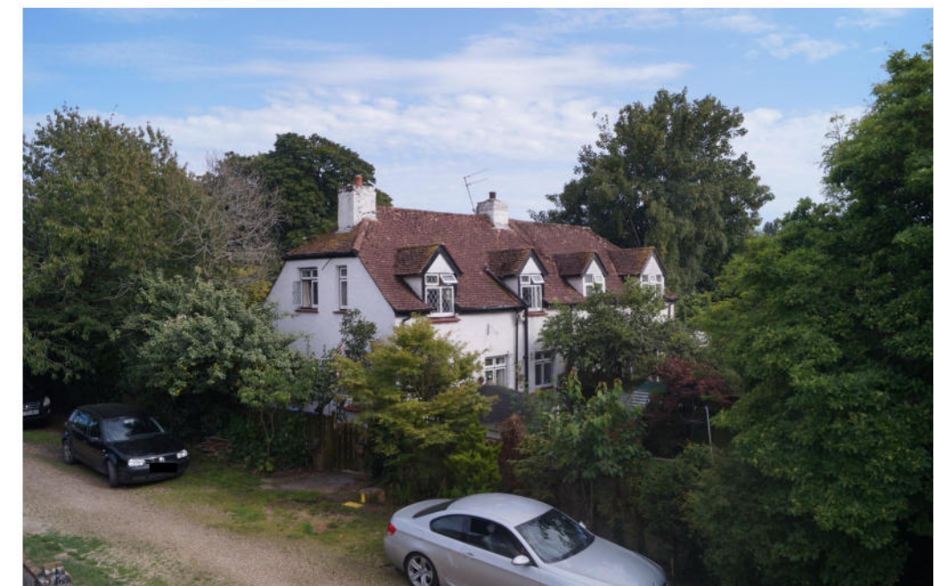
Fig. 9 View of The Barn and Barn Cottage—South of Barn End
