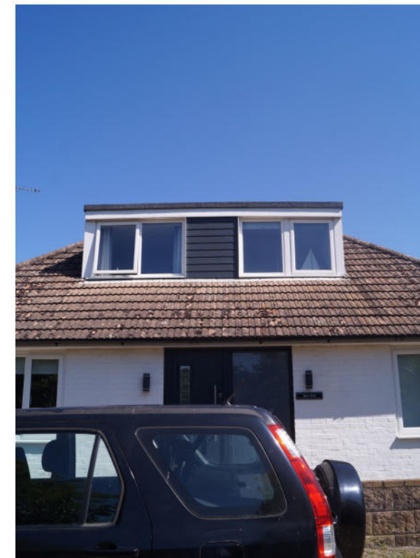
Fig. 2 Barn End - Front View
