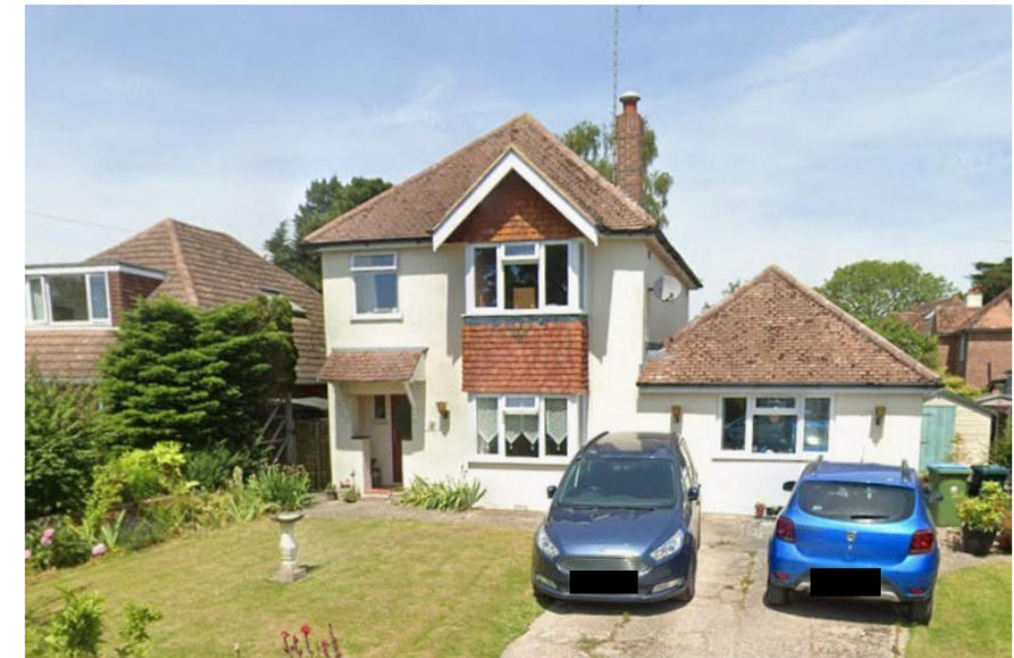
Fig. 6 View of The Owls—First House on North of Barn Lane
