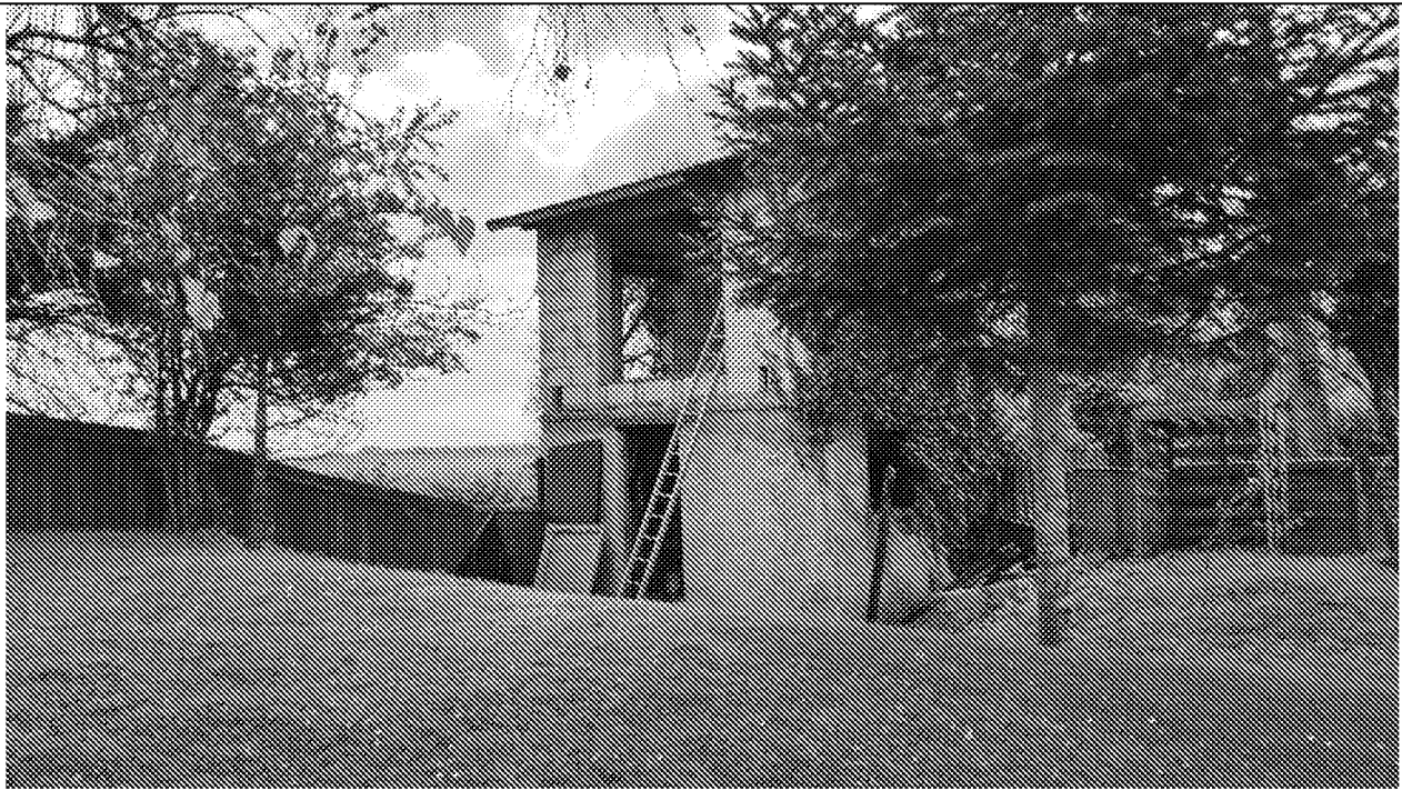
Photograph of concrete outbuilding in the south eastern corner of the site
