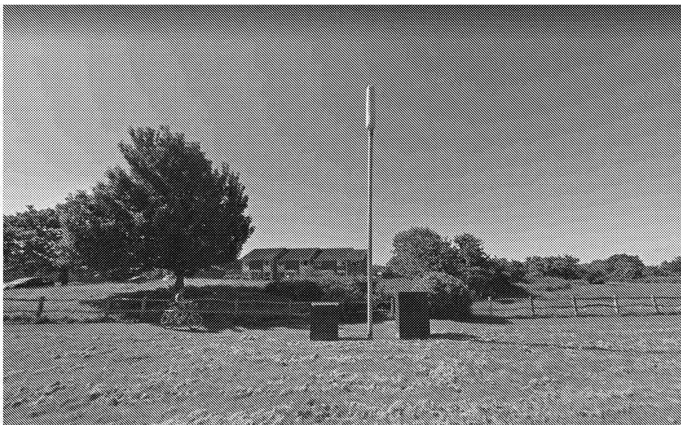
Image 1: Existing 2G/3G/4G site
