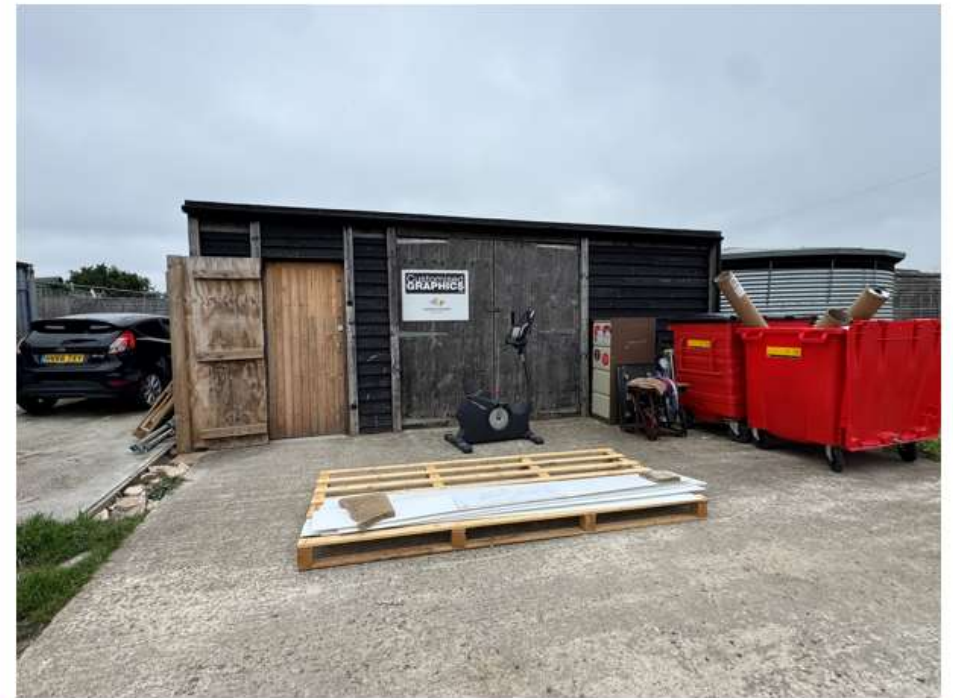
Photo No.12: Facing north showing vehicle graphics and glass repair and replacement unit in the centre of site
