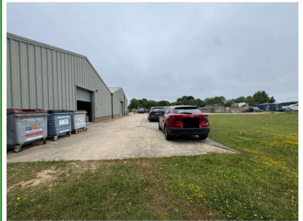
Photo No.20: Facing south showing the western face of the offsite industrial units located north of centre of site
