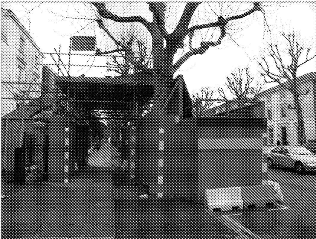
Picture 6: Where trees are off site, or public access is required through the work zone, boxing around the tree may be feasible.
