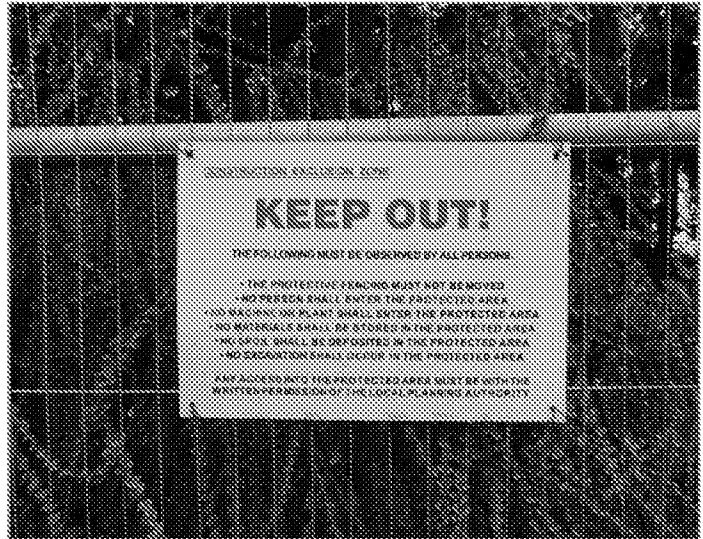
Picture 1: All barriers should be labelled to keep working activities outside the Construction Exclusion Zones (CEZs).
