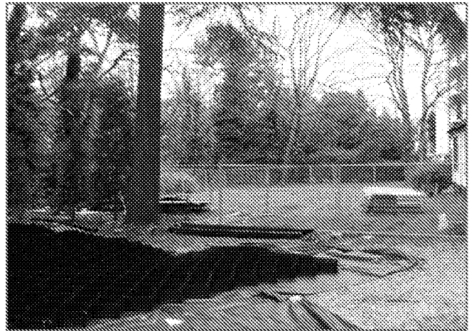
Pictures 3 and 4: Ground protection can be erected on scaffold platforms or with cellular confinement systems that can be easily lifted once the development has been completed
