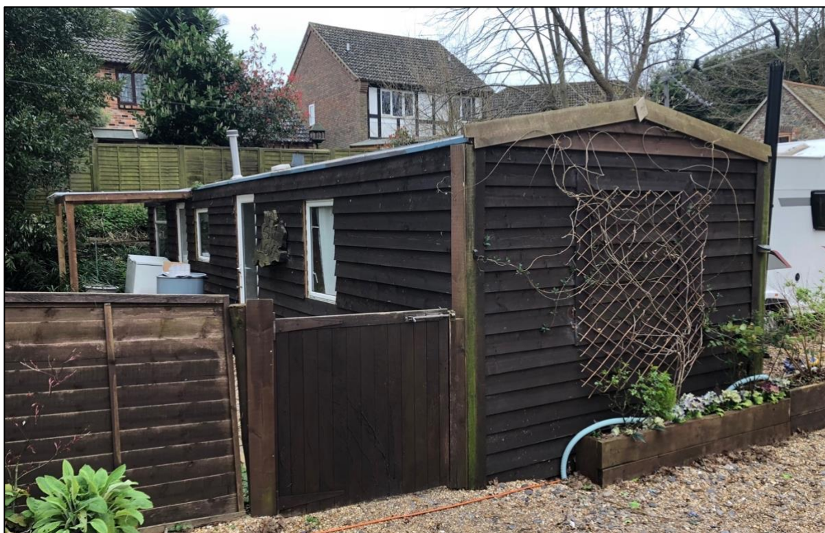
Photograph 7. The static caravan which is clad in wooden weatherboarding.
