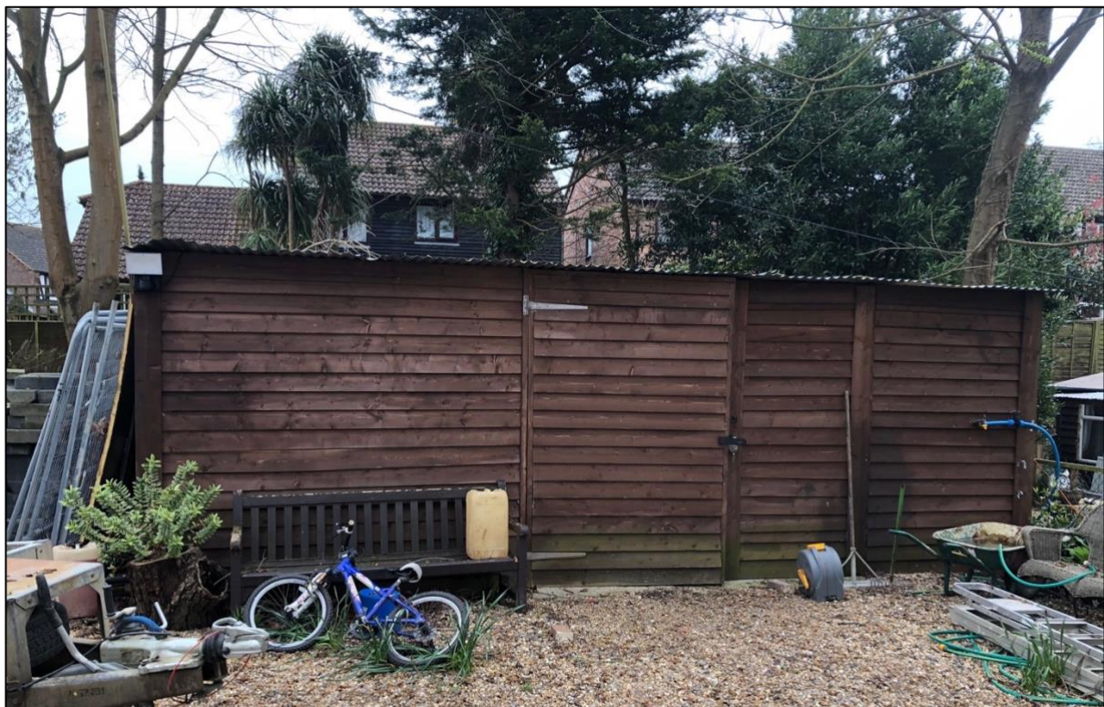
Photograph 5. The north-western elevation of the shed.
