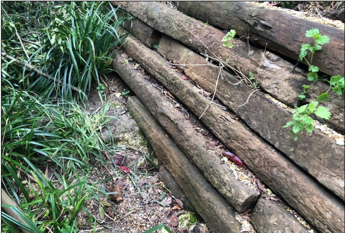
Photograph 15. Railway sleepers located behind the caravan. These have been used to reinforce the site's raised bank at the south-eastern boundary and create suitable sheltering/hibernating opportunities for amphibians including the great crested newt.
