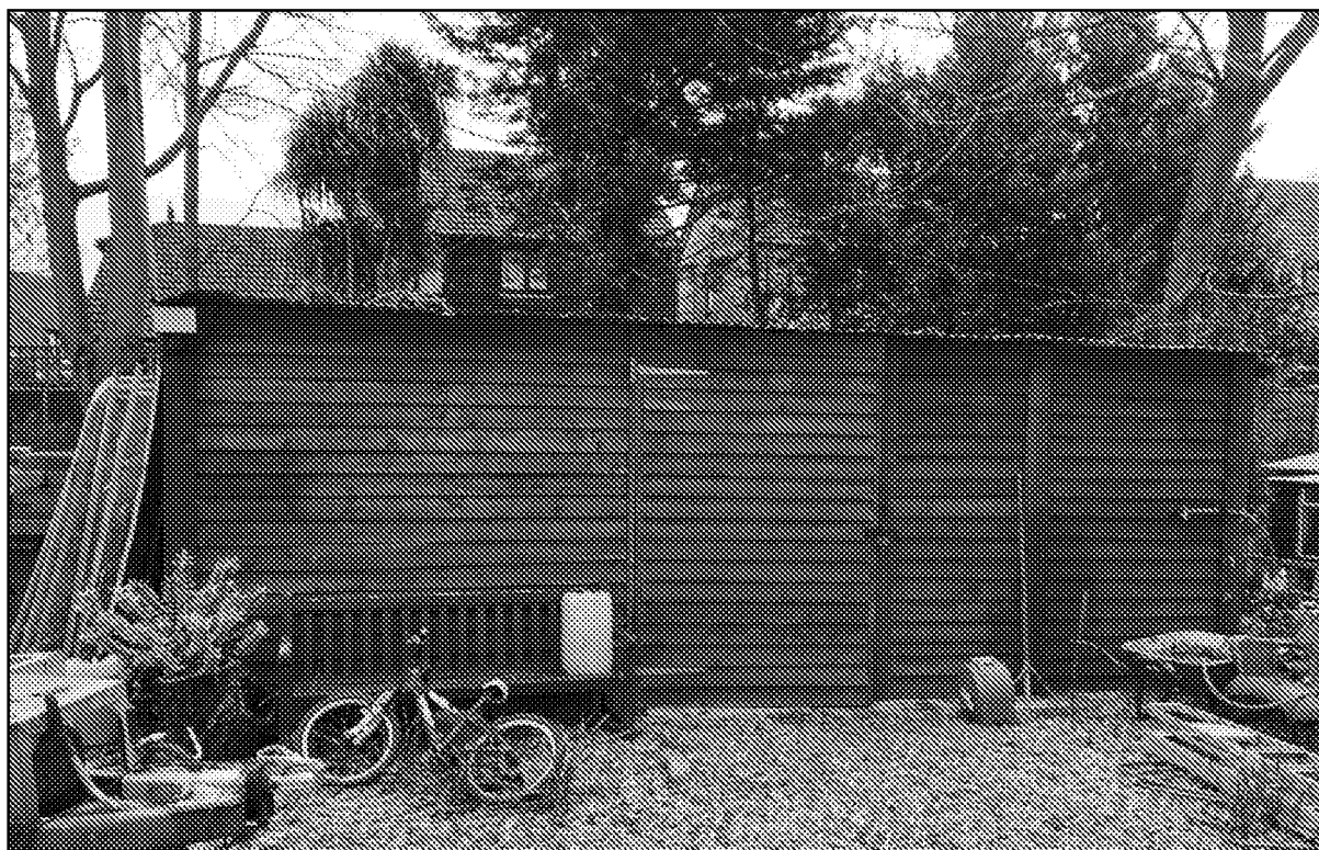
Photograph 5. The north-western elevation of the shed.
