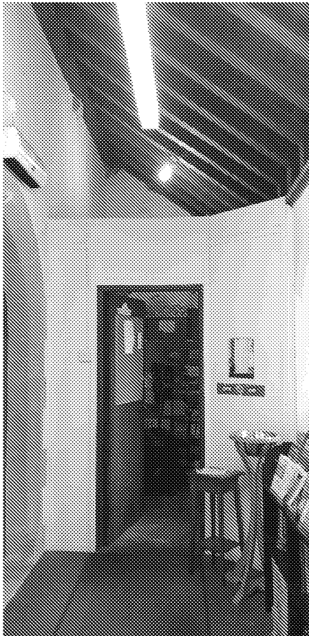
The existing storage room
