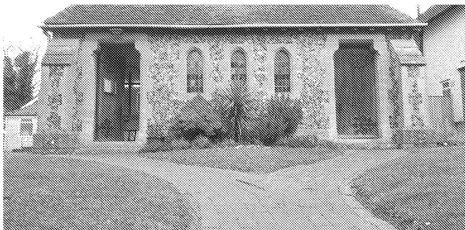
The existing split path and landscaping to the church entrance
