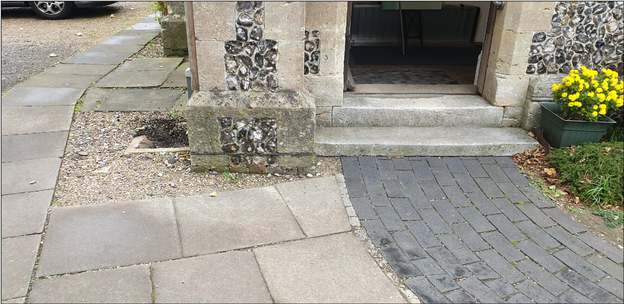
Stone Step Threshold and Paths near the Main Church Entrance
