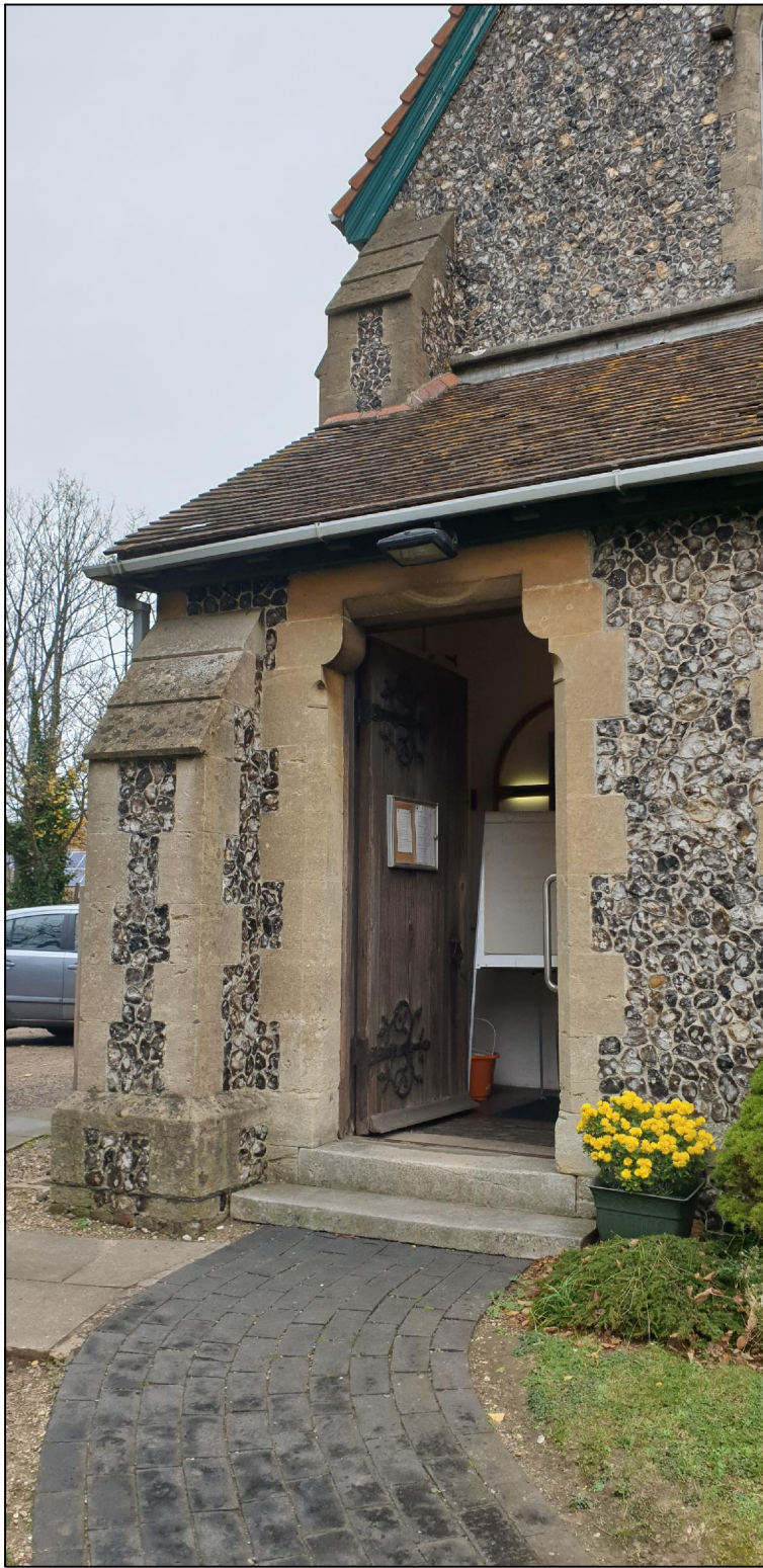
Main Processional Entrance
