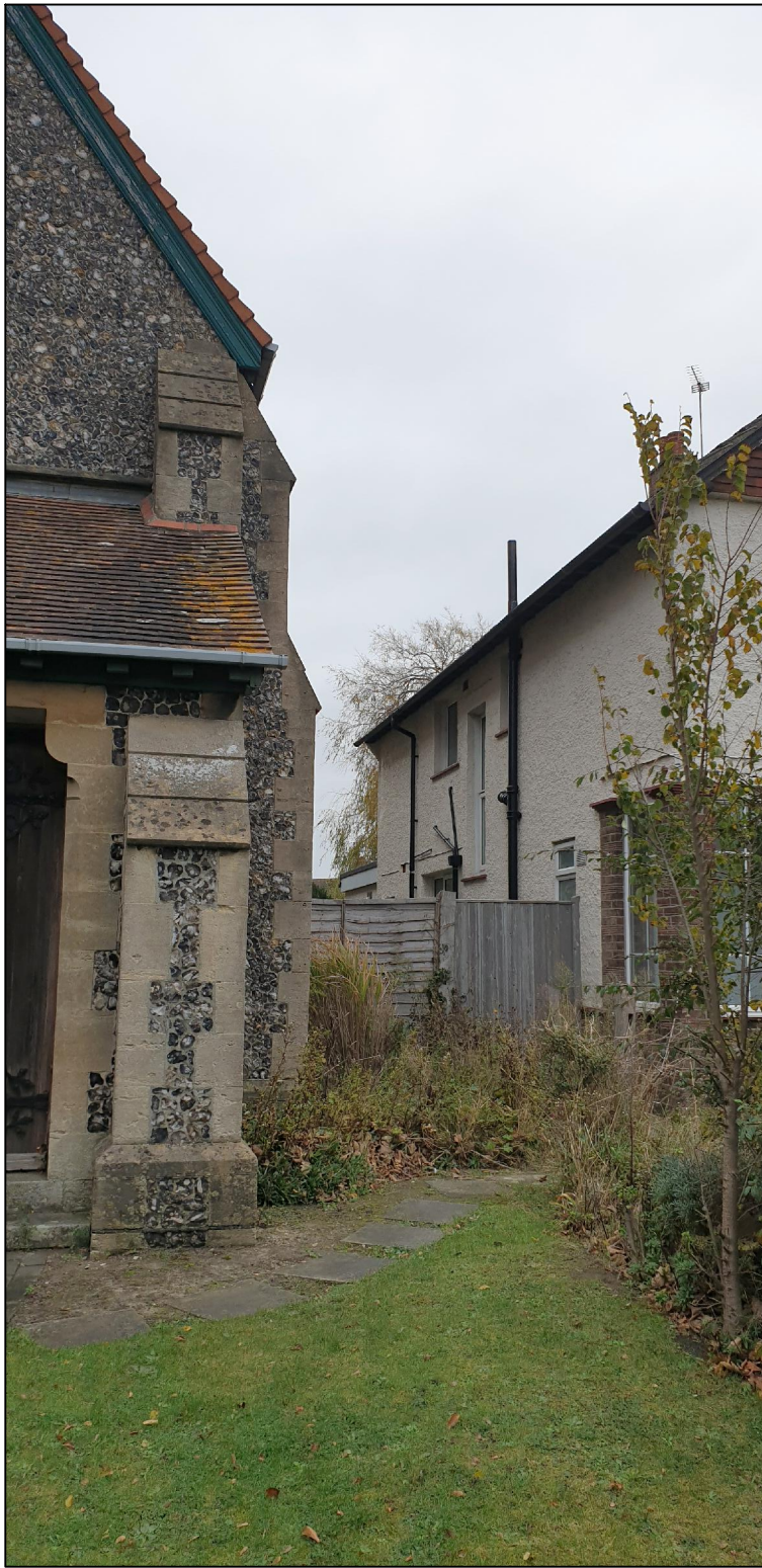
View of Eastern Boundary with Neighbouring Property
