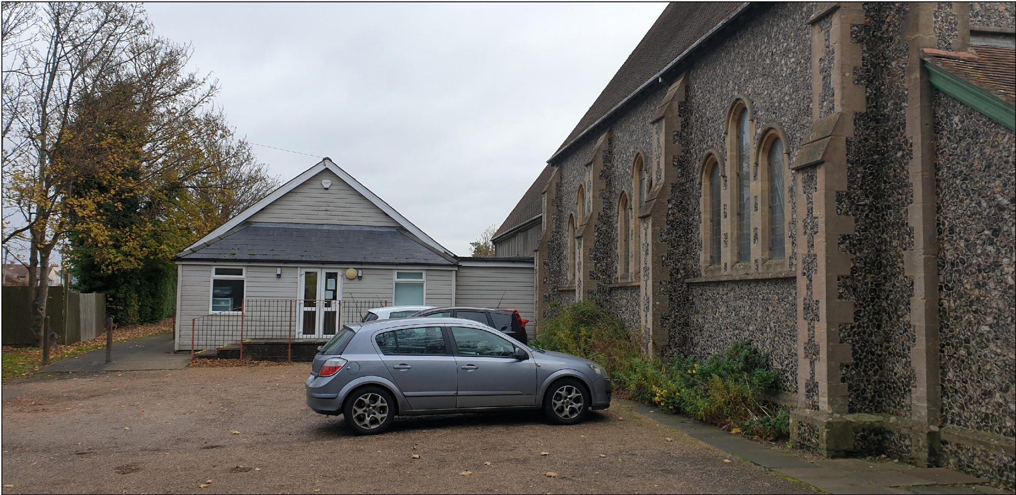
Community Hall and Car Park adjacent to the Church
