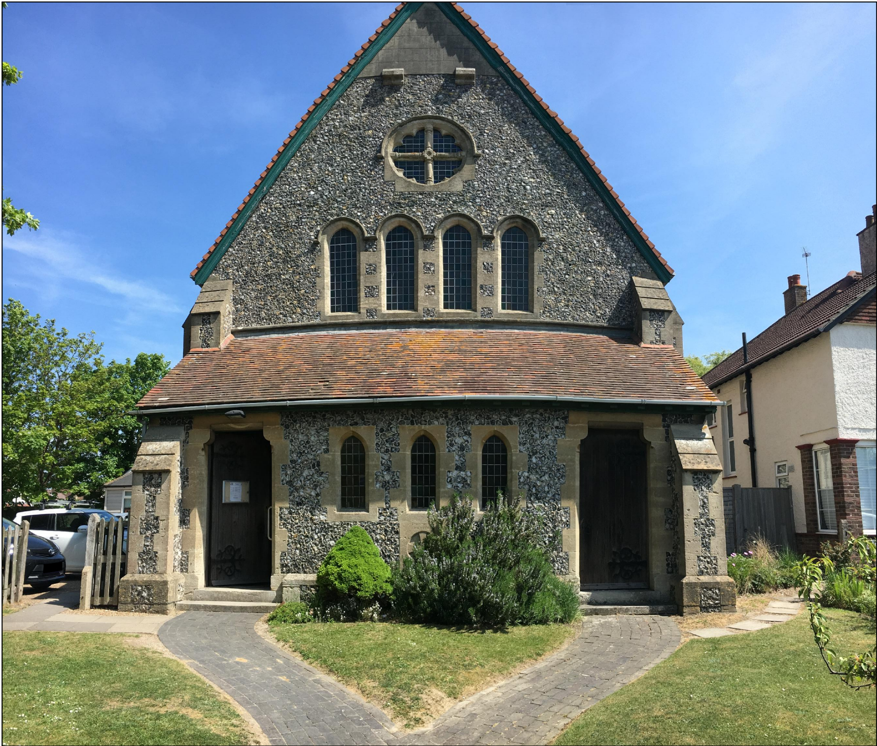
View of South West Elevation and Main Church Entrance
