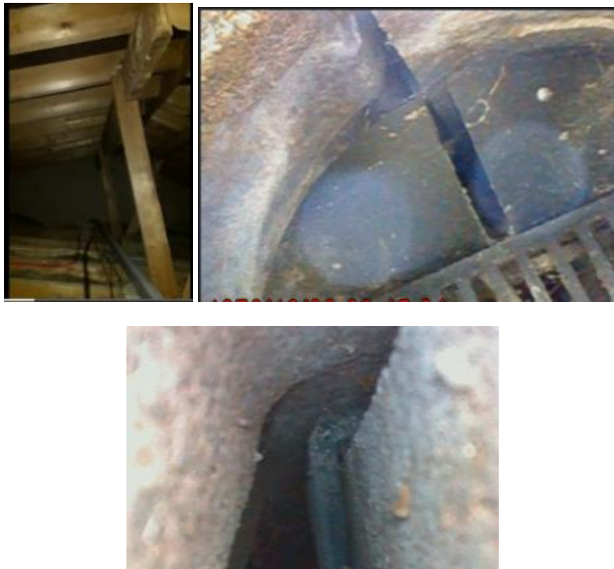
Figure 2: Showing the interior of the pitched roof section and two pictures of potential roost features in the external tiles.
