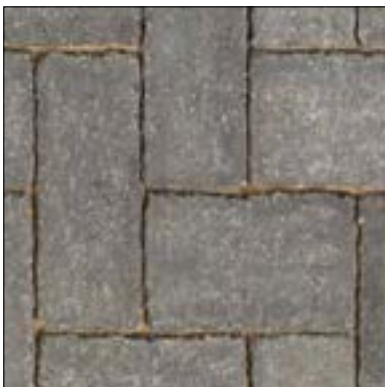
⑥ Concrete paving to road/footpath
