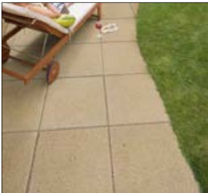
③ Concrete block paving to Patios
