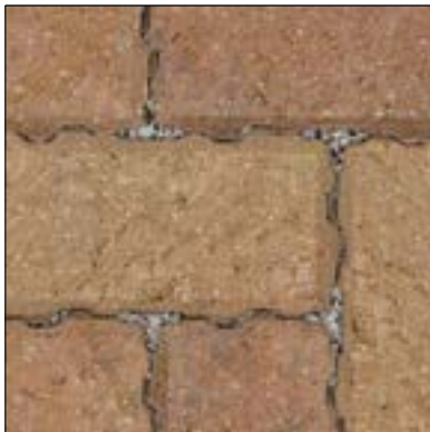
② Concrete paving to driveways
