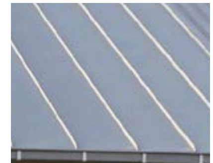
Zinc porch roof
