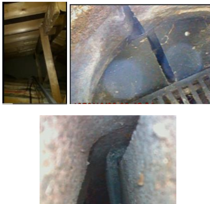
Figure 2: Showing the interior of the pitched roof section and two pictures of potential roost features in the external tiles.
