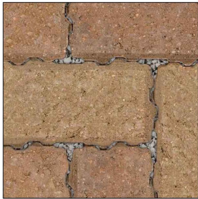
② Concrete paving to driveways
