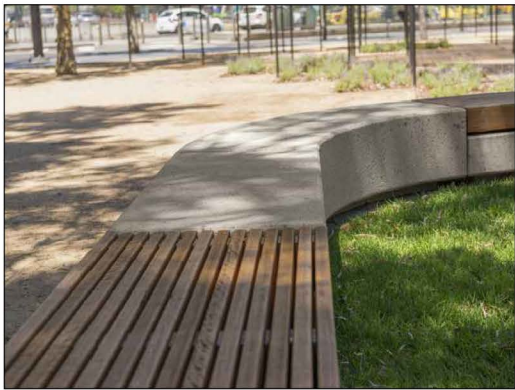
⑪ Curved Concrete Seating Wall
