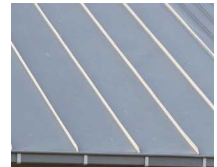
Zinc porch roof
