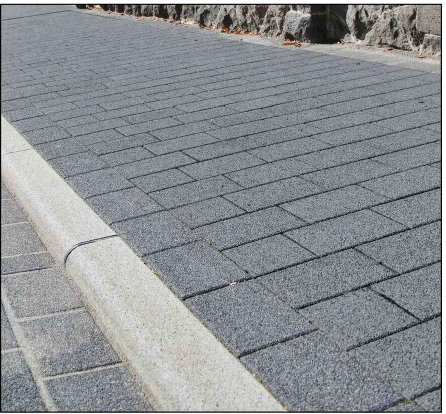
5 25mm upstand kerb - PCC Colour: Silver grey. Kerbs location as shown on 1444-HED-DR-02-002
