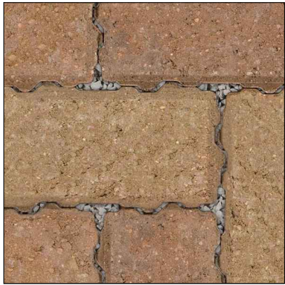
2 Concrete paving to driveways Product: Marshall Priora Permeable - Staggered bond Colour/ Finish: Bracken Size: 200 x 100 x 80mm
