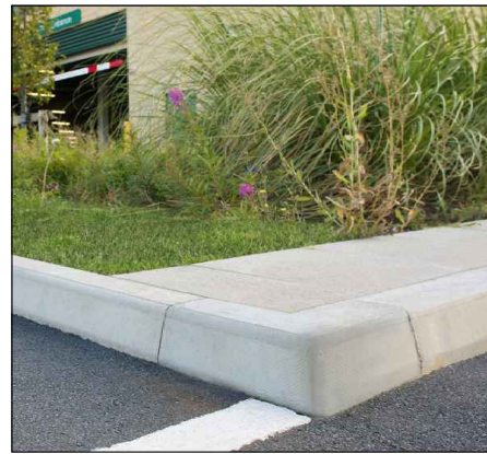
7 Standard kerb - PCC Colour: Silver grey. Kerbs location as shown on 1444-HED-DR-02-002
