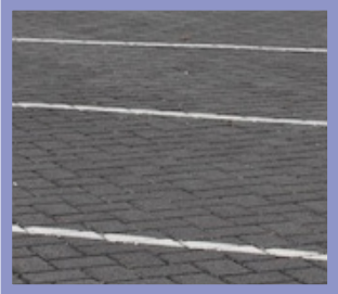
< Permeable block paving
