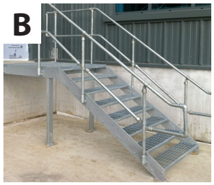
< Metal escape stairs
