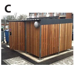
Timber clad bin storage >
