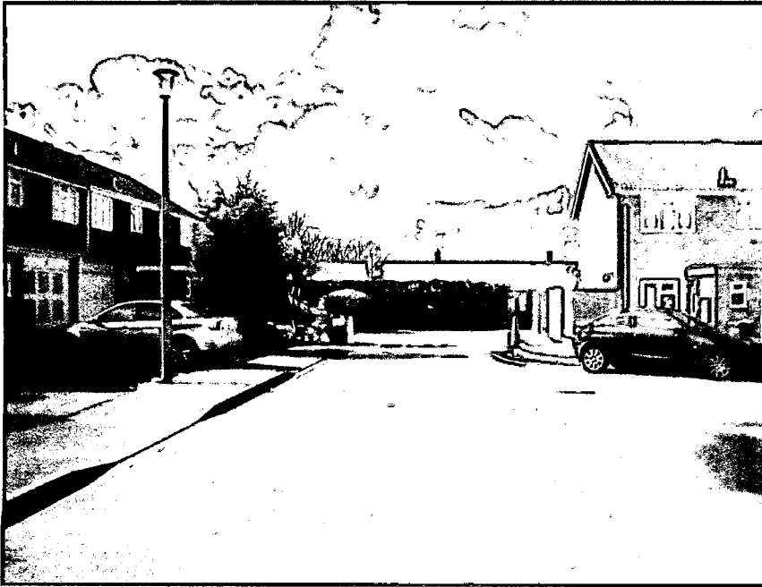
Ashurst Close Entrance to No 11
