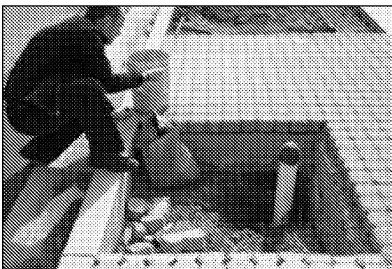
Photo 57: The finished surfacing is profiled to leave the tree pit open, ready to be filled with good quality topsoil and the new tree.
