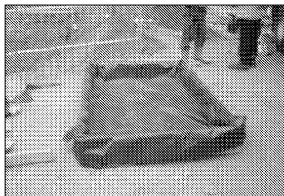
Photo 47: Soil bunding or a supporting framework covered in heavy-duty plastic sheeting is essential where there is a risk of spillages contaminating RPAs. This specifically applies to
