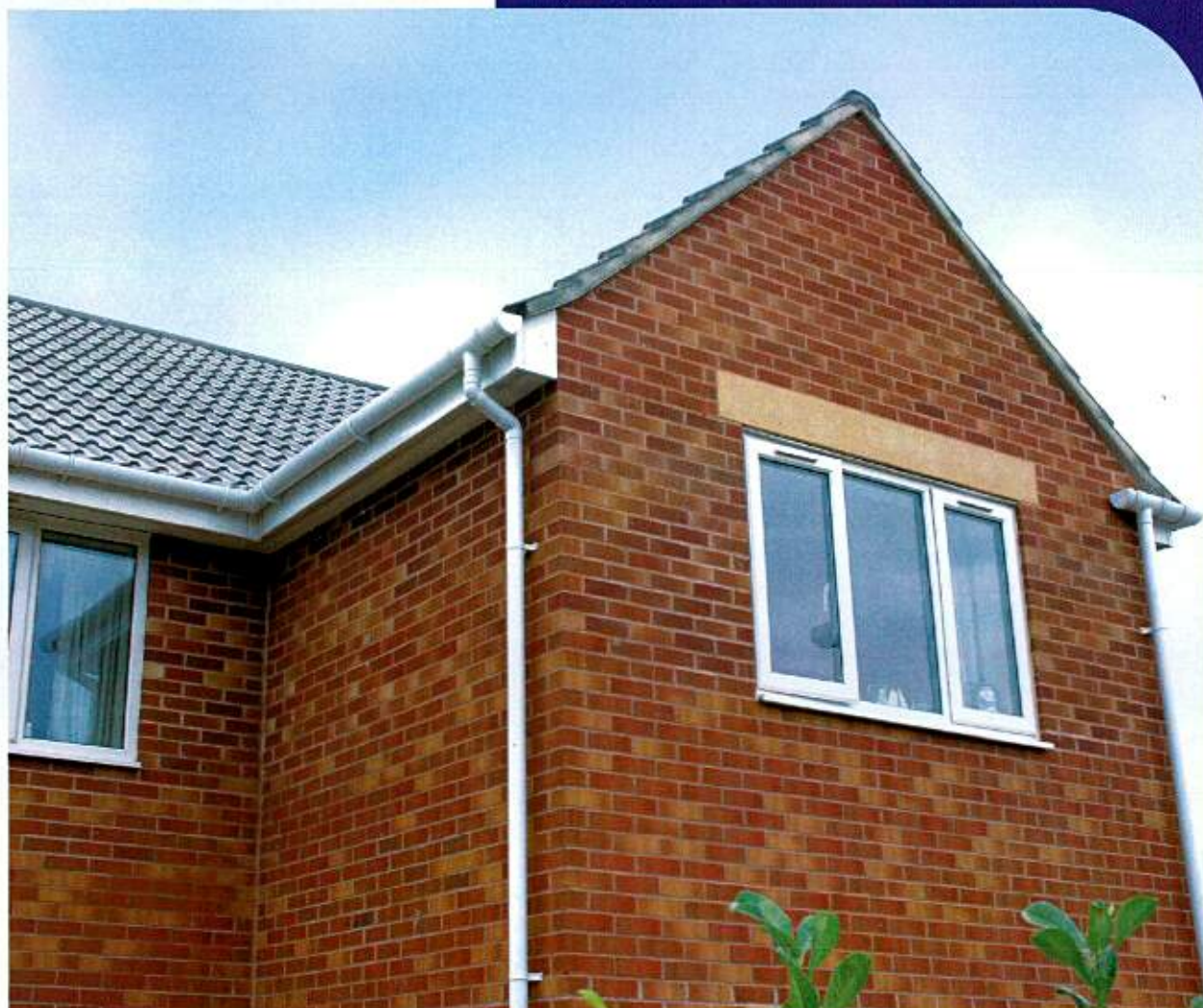
Private House, Dursley, Gloucestershire
