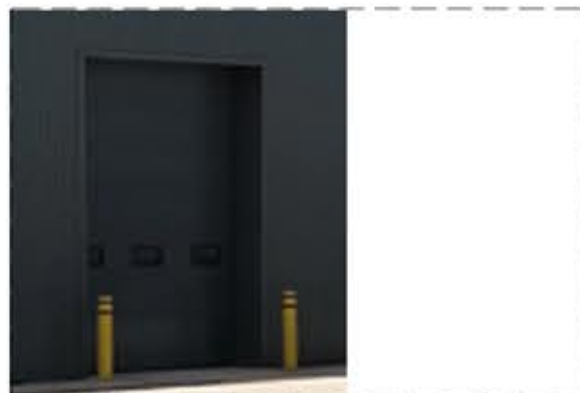
M Sectional vertical lift level access loading door Size: 4000mm wide x 5000mm high (clear opening) Colour: Grey White (RAL 9002)
