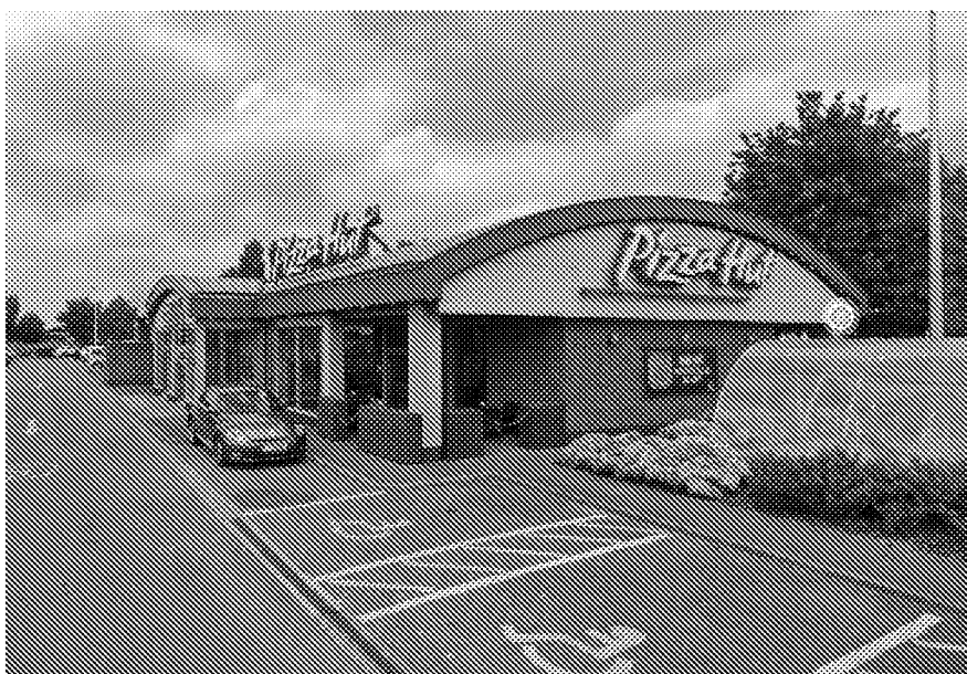
Photograph 1. Existing pizza hut building
