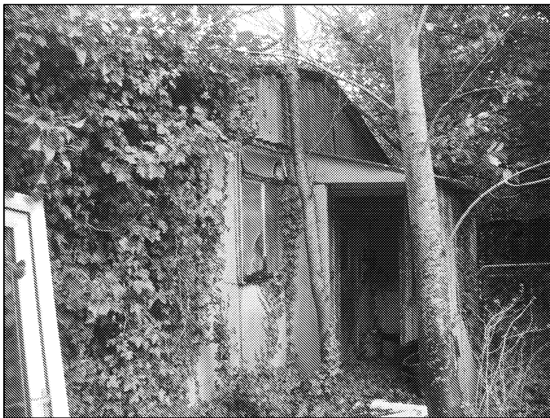
Photo 9. Showing the entry porch on the southern elevation of building 3.
