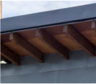
> 10 - Treated timber rafters
