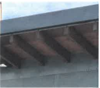
< 6 - Treated timber rafters
