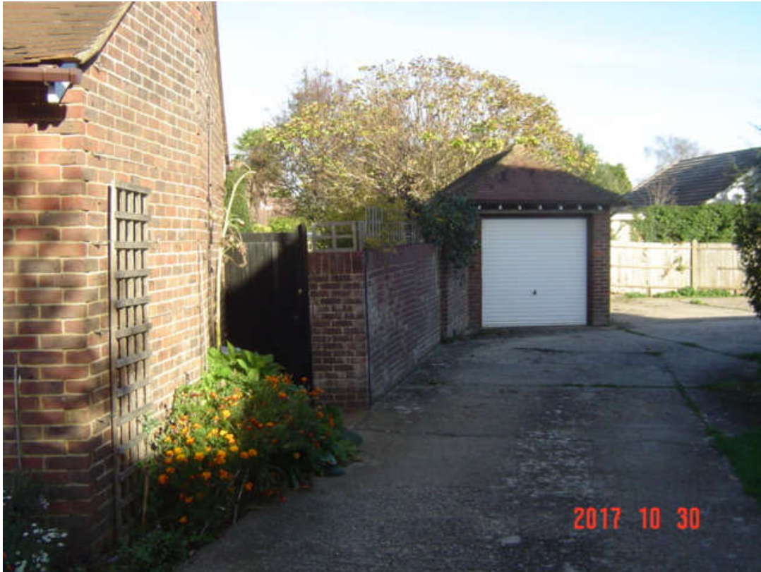
View from Homing Gardens of garage and access road
