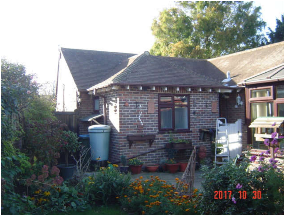
Exterior of en-suite, location of kitchen extension
