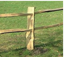
Proposed fencing to the front garden plots 1-6 - Chestnut cleft fencing
