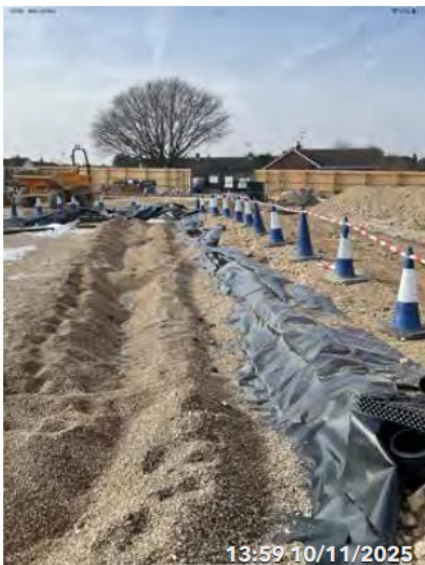
Swale On The outside of The Attenuation Tank Assigned To Lovells Membrane laid out to the kerb, shingle fill. .100mm land drain wrapped in terram,
