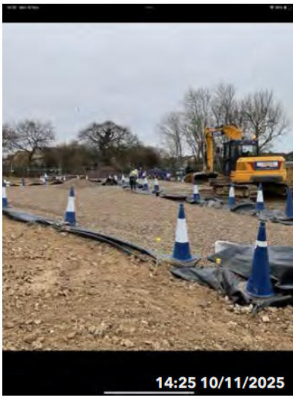
Swale Outside Of The Attenuation Tank Assigned To Lovells Back fill over the wraparound. Level with stone.
