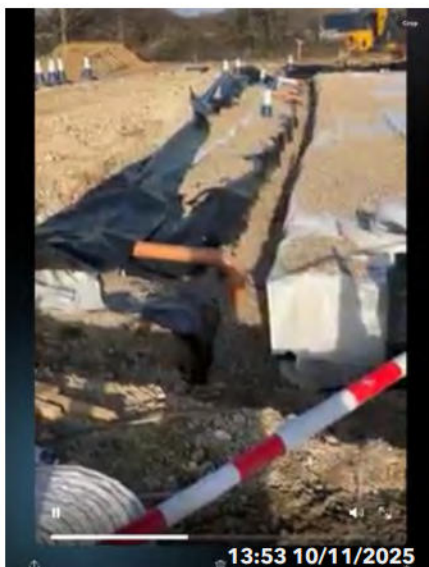
Swale On The outside of The Attenuation Tank Assigned To Lovells Membrane laid out to the kerb, shingle fill.
