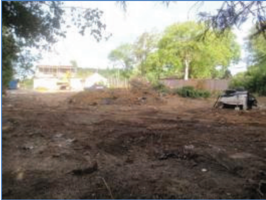
Plate 1: Pre-excavation, from the east
