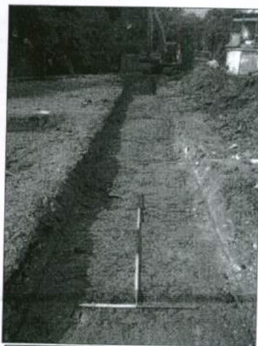
Plate 8: Trench 3, from the north-east
