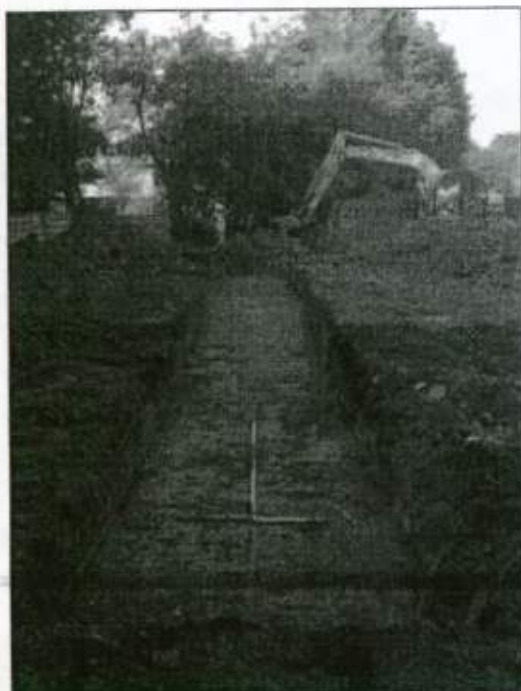
Plate 2: Trench 1, from the north-east
