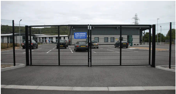
Vehicular entrance gates
