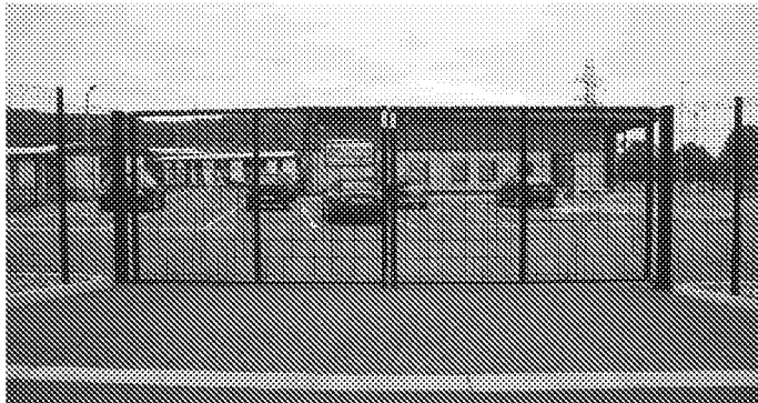
Vehicular entrance gates
