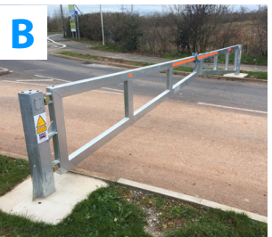
1m Car park barrier (White PPC finish) (closed out of hours) >
