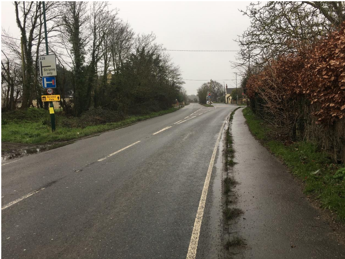
Southbound approach along the A29 to the proposed informal pedestrian crossing
