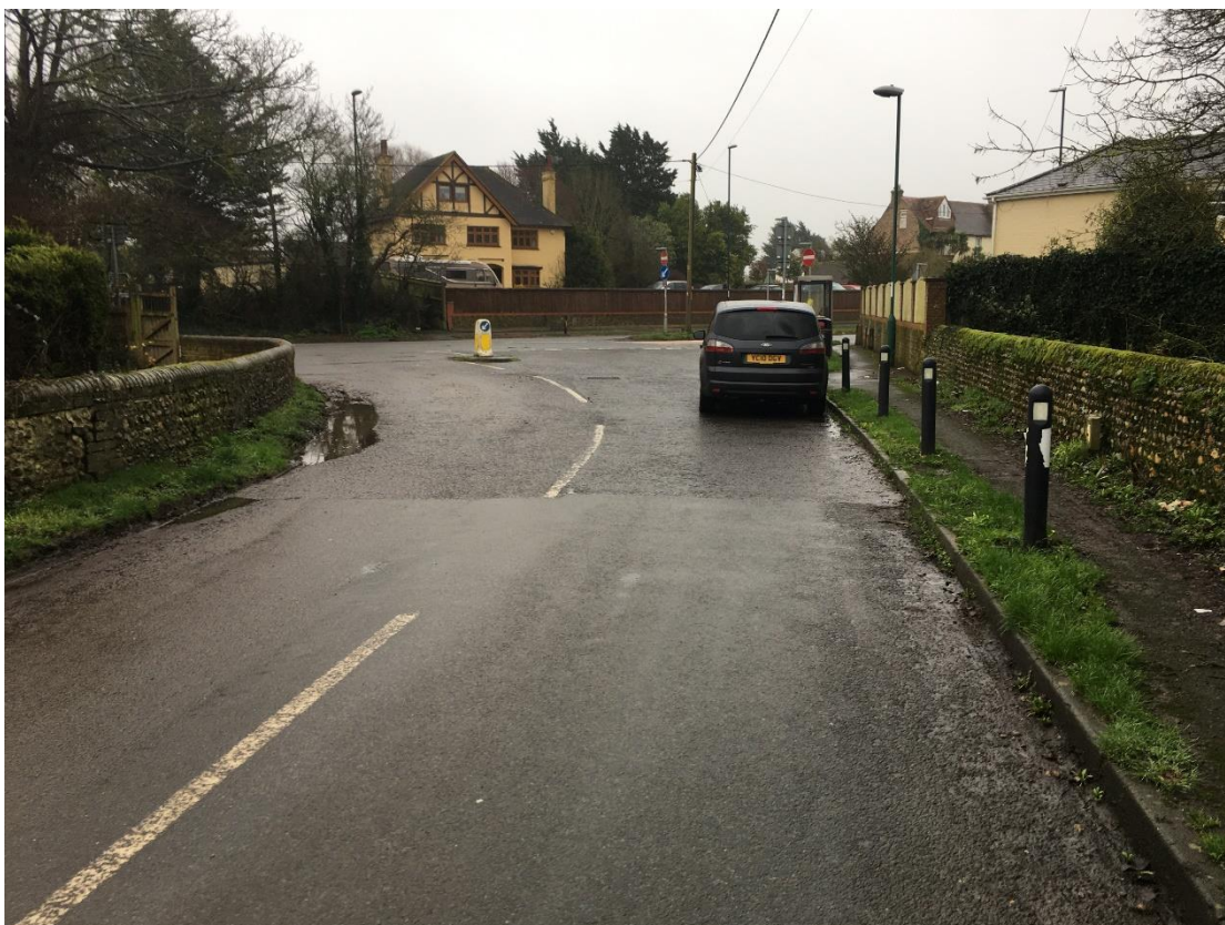
Eastbound approach to the A29 along Shripney Lane
