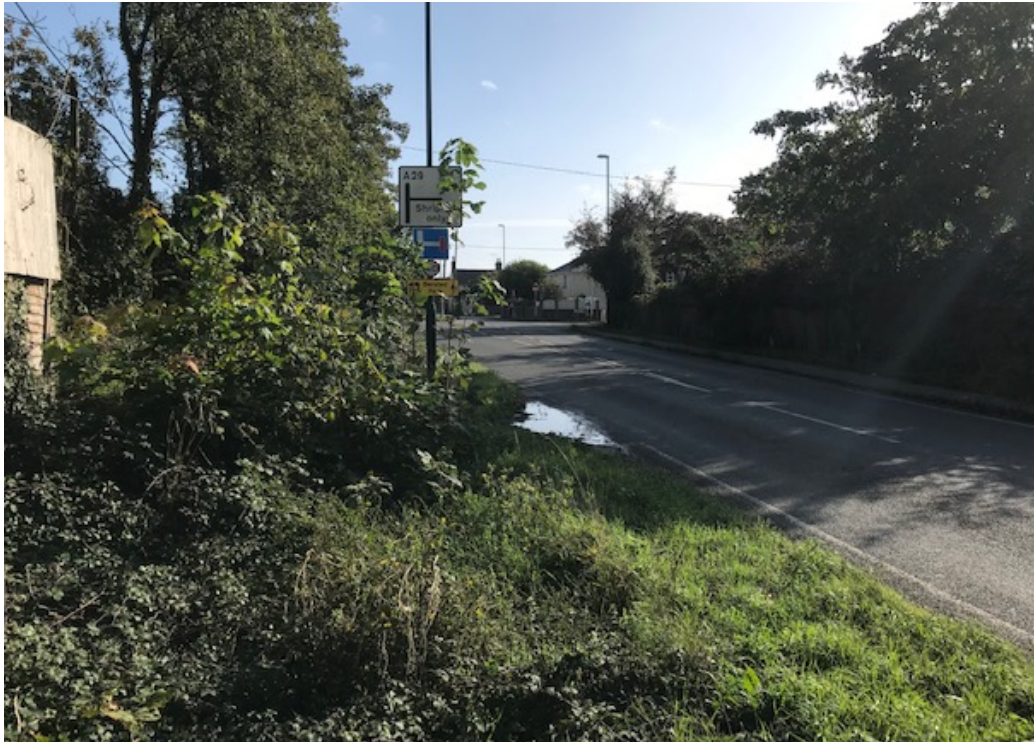
Photo 2.1a Visibility to the south of the proposed junction is obscured by vegetation
