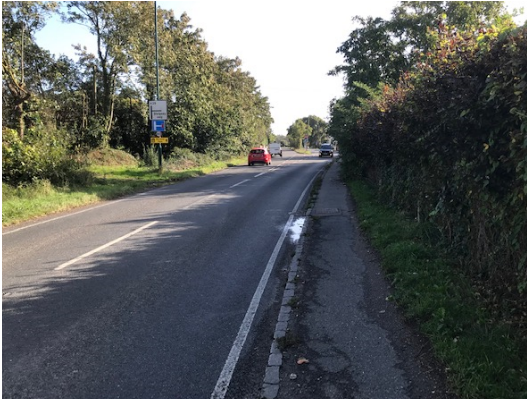
Photo 2.4 - Visibility for pedestrians using the proposed crossing facilities will become obscured if vegetation is not maintained
