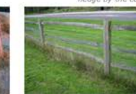
Hardwood post and rail fencing
