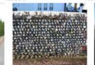
Flint wall with half round brick coping
