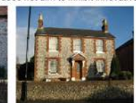
Flint cottage with slate roof
