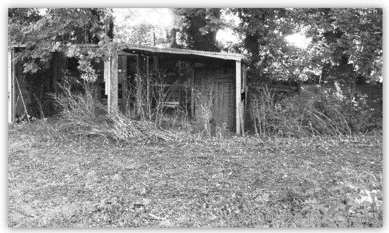
Photograph 2. Open fronted timber structure.
