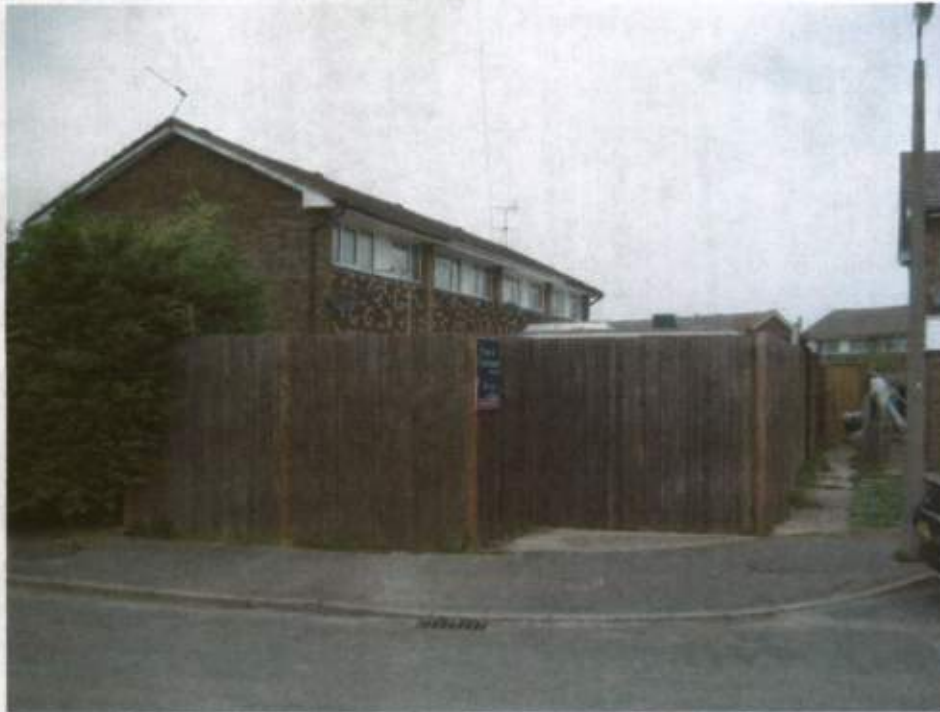
The proposed location for the garage as viewed from the road
