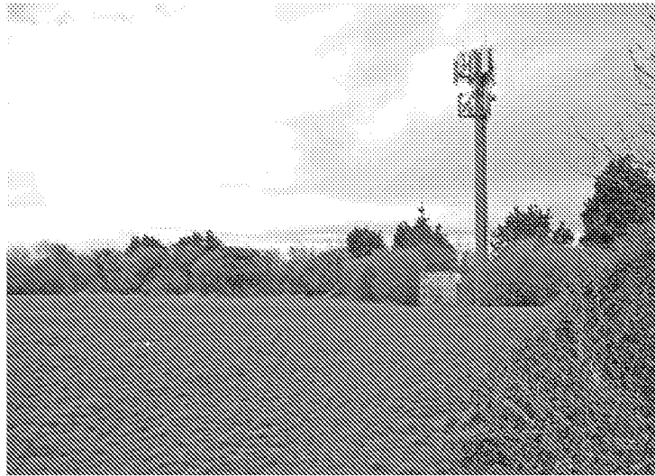
9. MOBILE NETWORK TOWER
